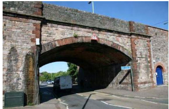
Here the abutments look solid.
