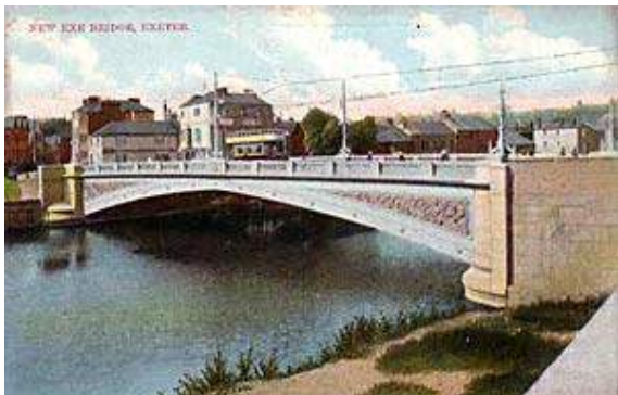
The flood pressures would be eased considerably by the 1905 single span bridge. It is an interesting
