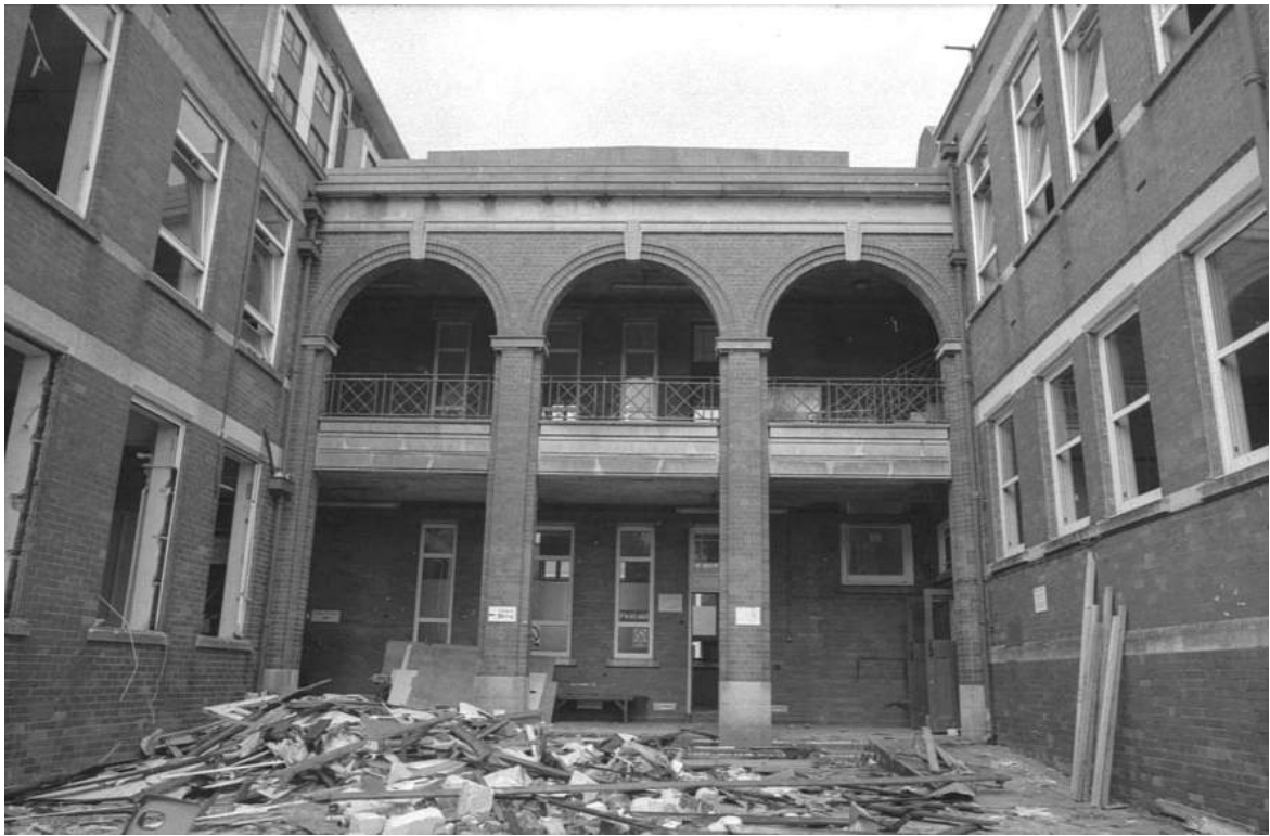
Fig.7 & 7a The 1931 building and loggia by John Bennett at Hele's School in August 2005, during the stripping of the building prior to demolition.
