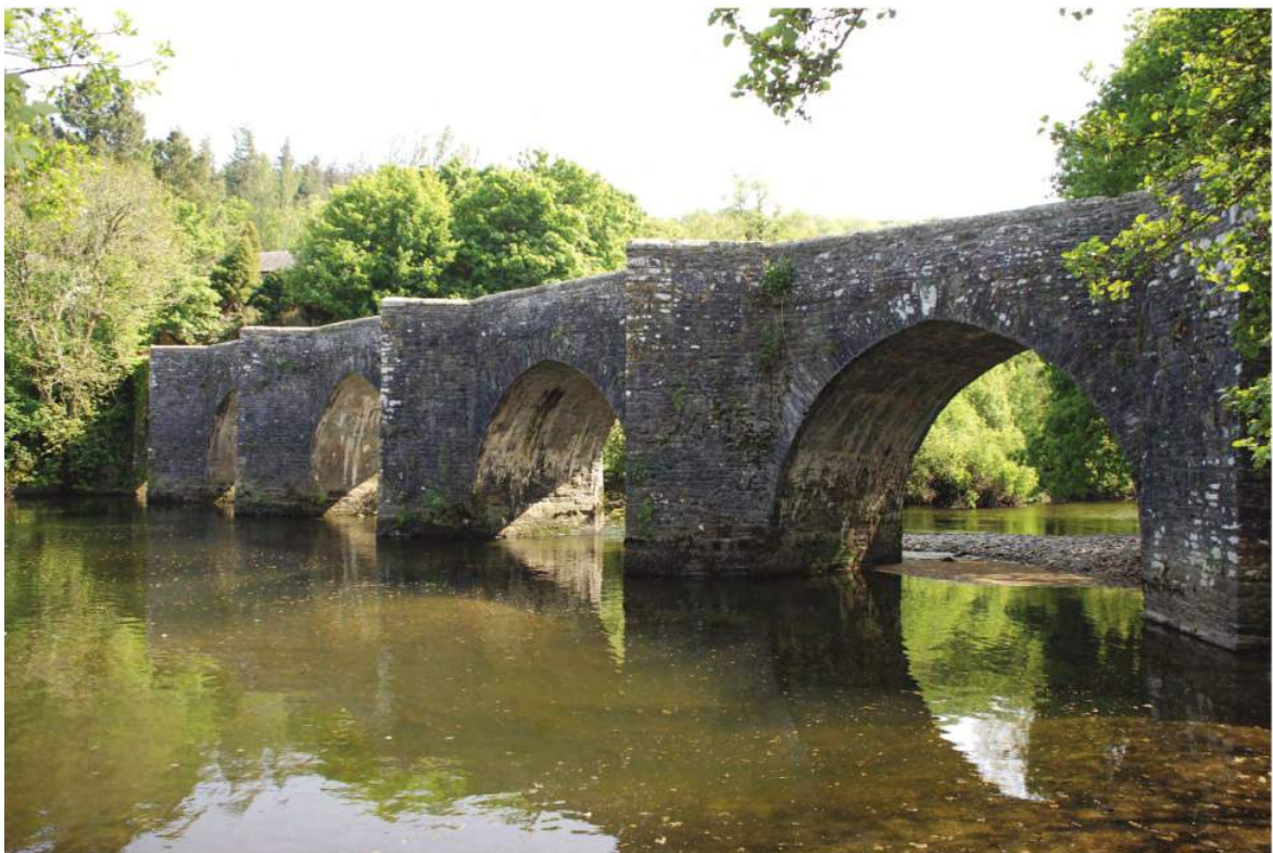
Fig. 17 Staverton Bridge, showing four of its seven pointed arches.
