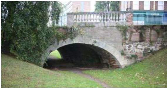
The one remaining span of the Georgian bridge shows a distinct lack of concern over skew.
