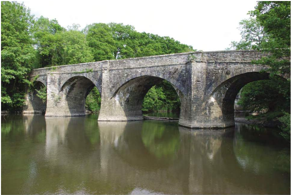
Fig. 16 Rothern Bridge, showing its four pointed arches which were widened in the post-medieval period.
