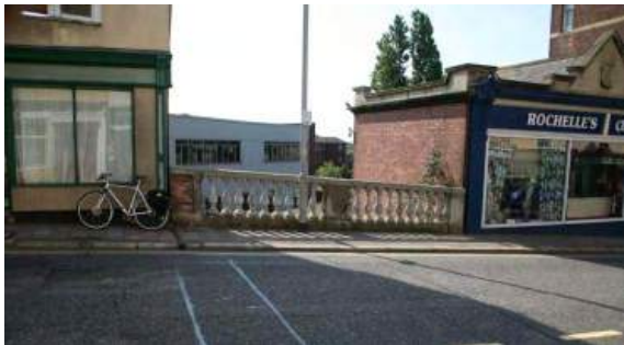
A very similar parapet to this appears in Fore Street where it crosses the mill leat. That crossing must be of a similar age to the new bridge. Is new bridge street between retaining walls or is it a hidden viaduct?
