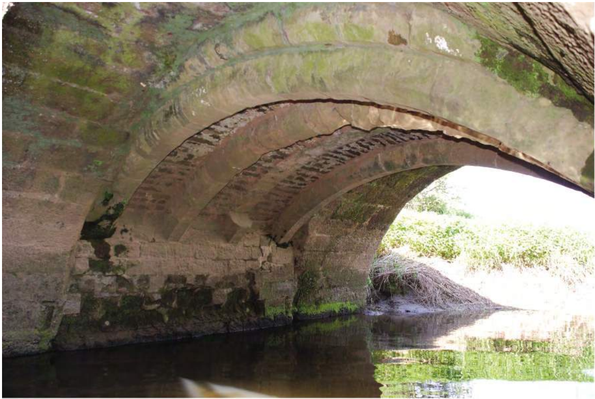
Fig. 8 Clyst St. Mary Bridge, showing one of two low segmental arches with narrow chamfered ribs.
