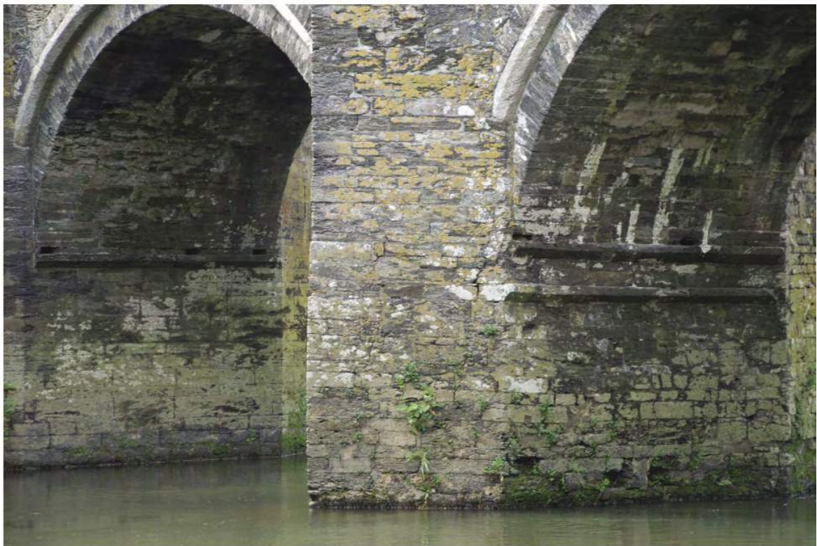
Fig. 23 Greystone Bridge, showing the two imposts beneath the central arch.
