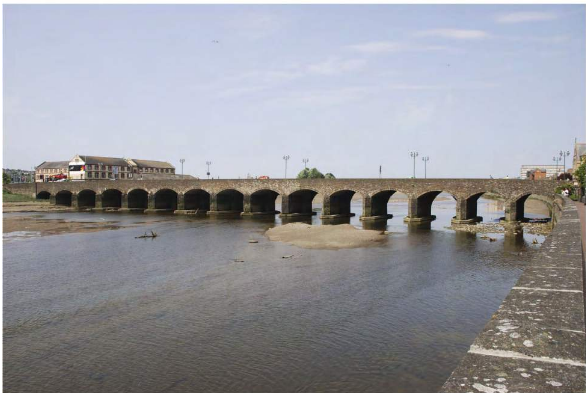
Fig. 13 Barnstaple Long Bridge, showing its sixteen pointed arches which were widened in the 18th and early 19th century.
