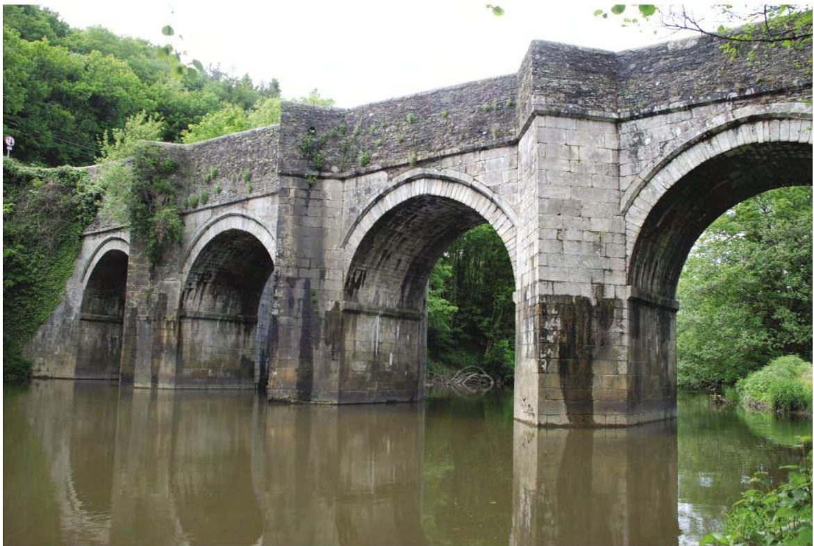
Fig. 19 New Bridge Gunnislake, showing the river arches dating from 1773.
