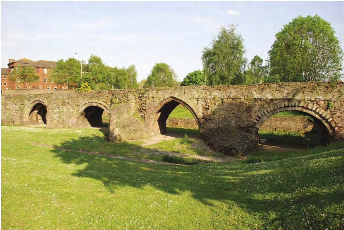
Fig. 1 The Medieval Exe Bridge, Exeter
