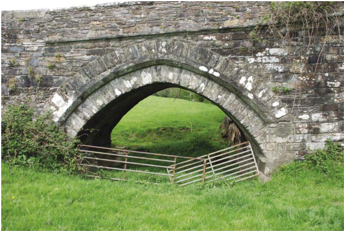
Fig. 20 Horse Bridge, showing the pointed land arch.
