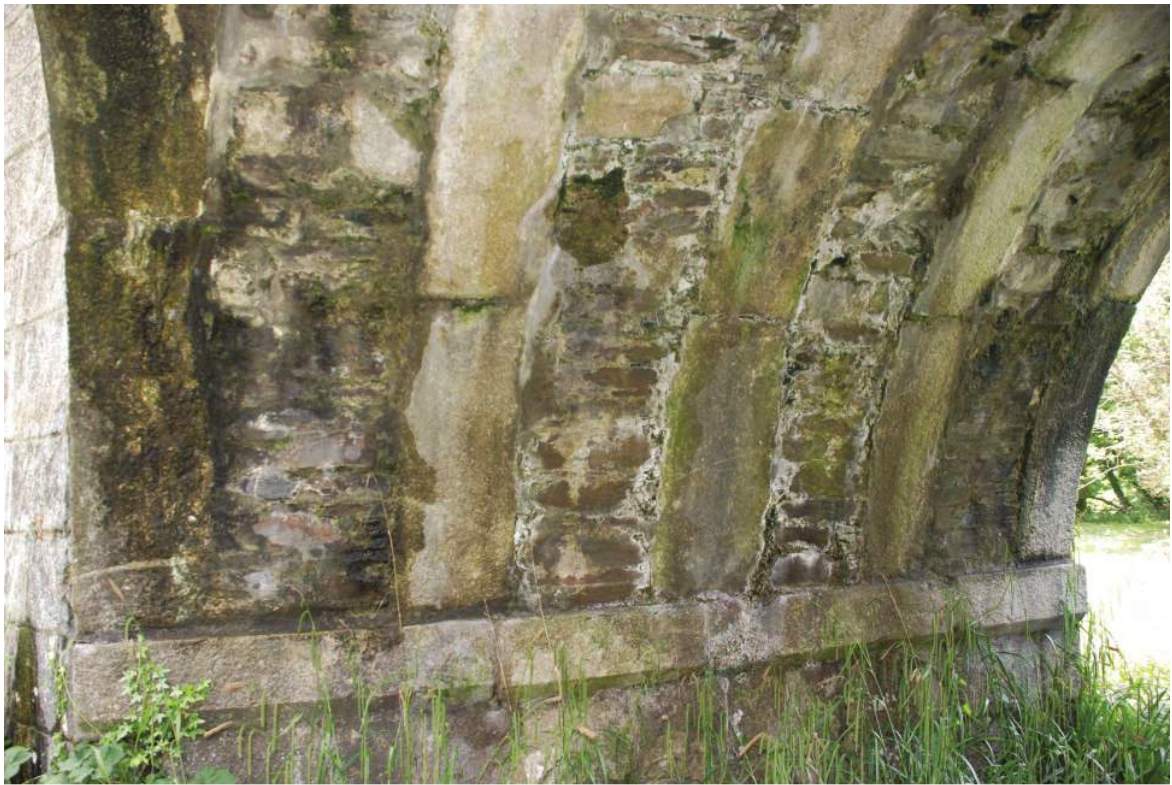
Fig. 18 New Bridge, Gunnislake, showing the ribbed land arch.
