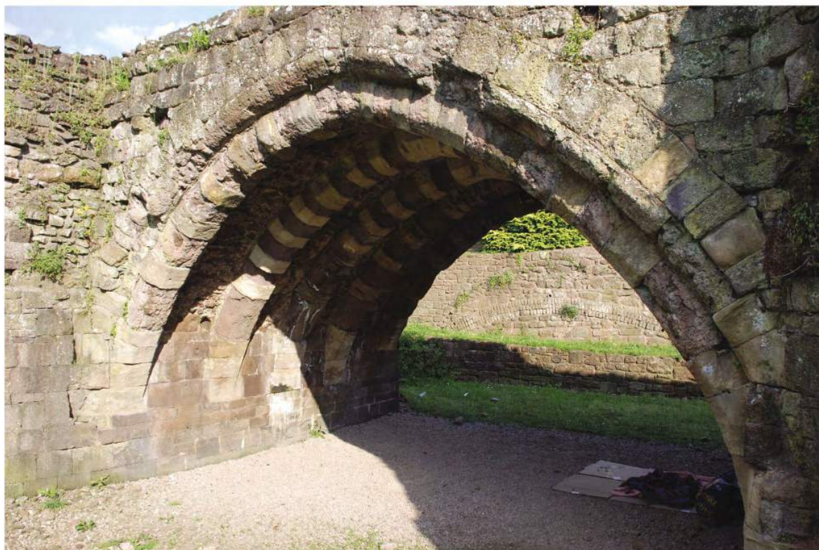
Fig. 4 Exe Bridge - a pointed arch showing narrow ribs with decorative alternating stone types and three arch rings, the lower two being chamfered.
