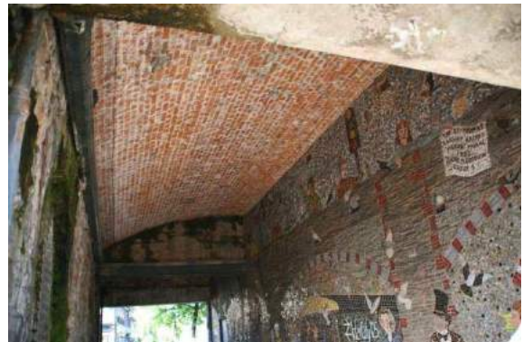
But look up in the footway and part of the arch is obviously hidden.
