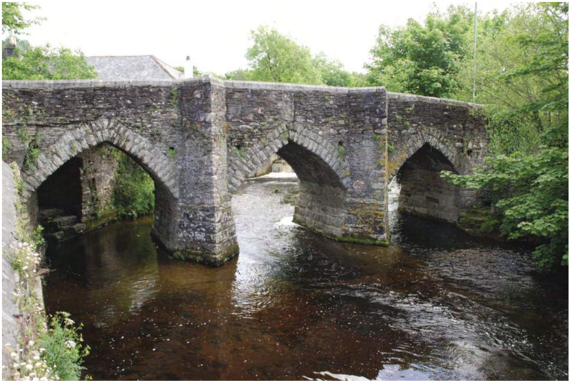
Fig. 14 Horrabridge Bridge, showing pointed arches similar to Barnstaple Bridge.
