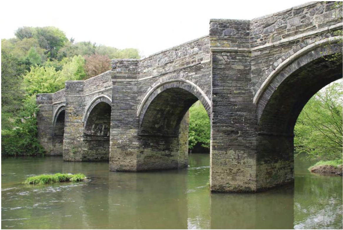
Fig. 22 Greystone Bridge, showing four of its five semicircular arches.
