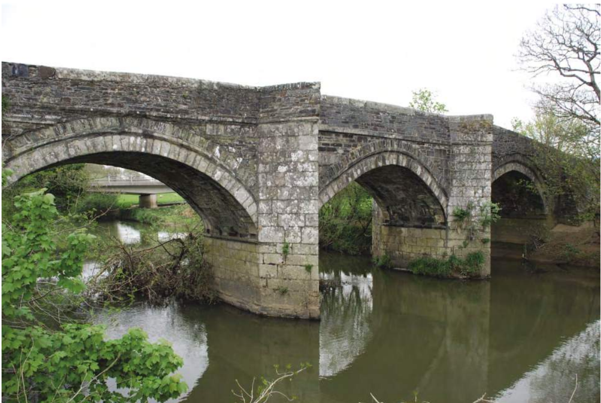
Fig. 25 Higher New Bridge, showing the three river arches.
