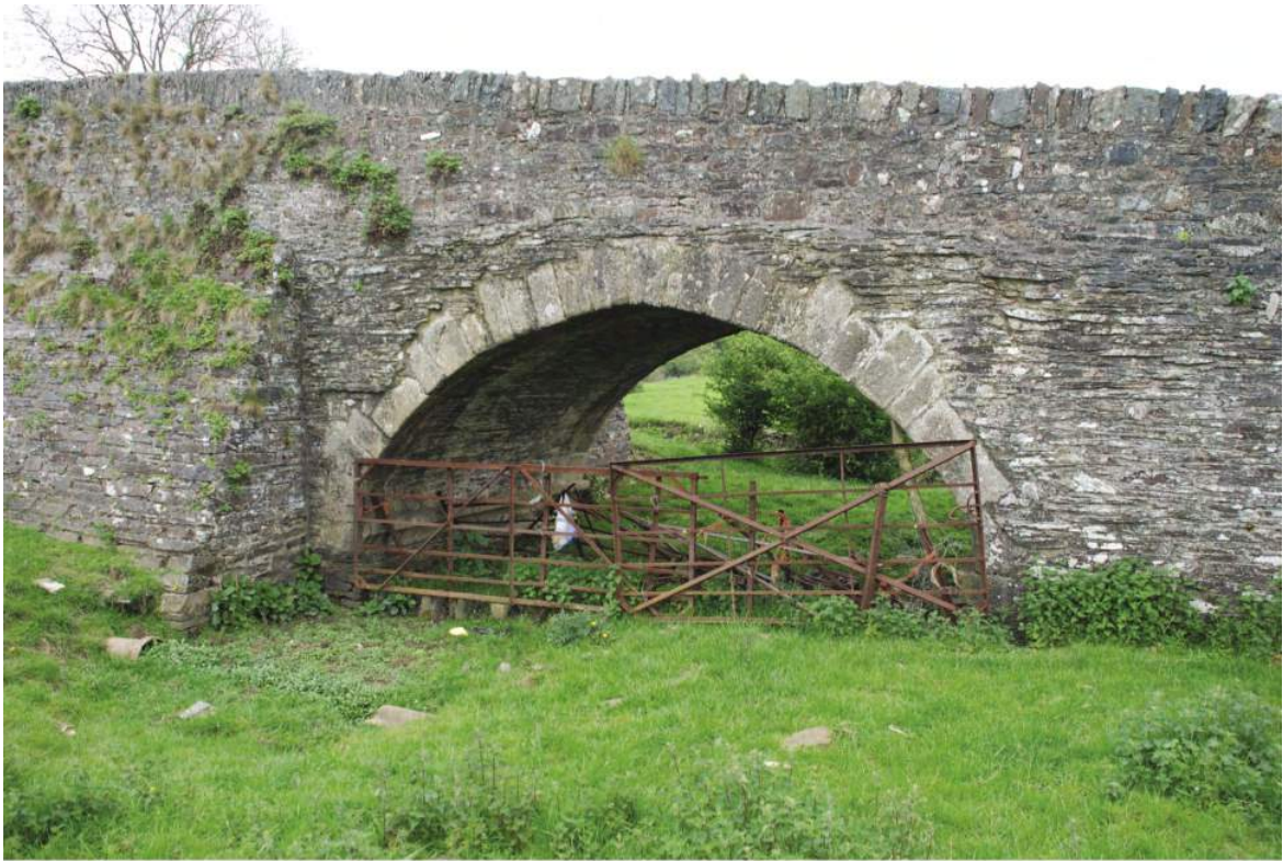
Fig. 24 Higher New Bridge, showing the land arch.
