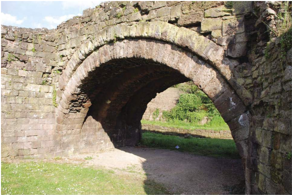
Fig. 3 Exe Bridge - a round arch, showing broad ribs and two arch rings.
