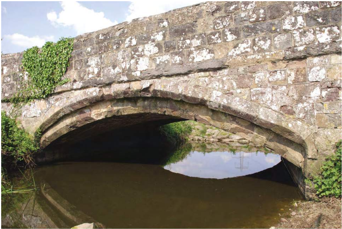
Fig. 10 Stoke Canon Bridge, showing the earliest low segmental arch which has no ribs.
