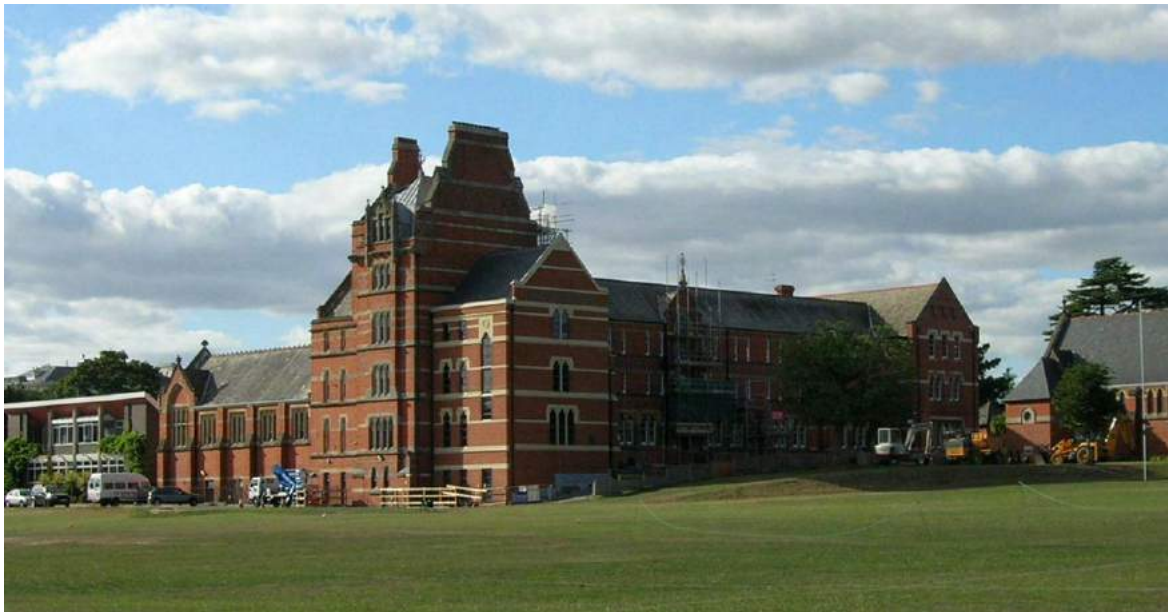
Fig.10 Exeter School, Victoria Park Road showing the new building attached to Butterfield's range of 1880, August 2006.
