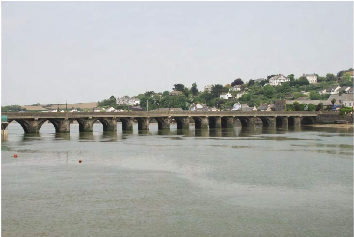
Fig. 12 Bideford Long Bridge, showing its twenty-four pointed arches which were widened in about 1820.
