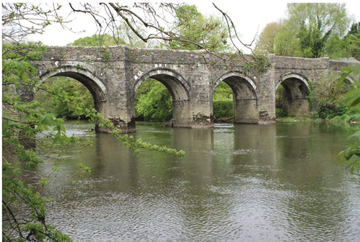
Fig. 21 Horse Bridge, showing five of the six round river arches of probable post-medieval date.
