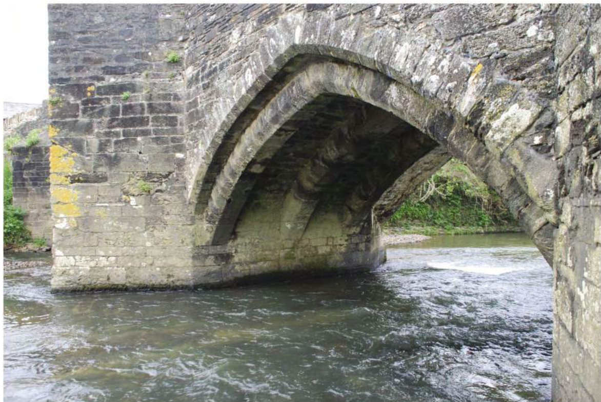
Fig. 9 Yeolm Bridge, showing one of two pointed arches with narrow chamfered ribs.
