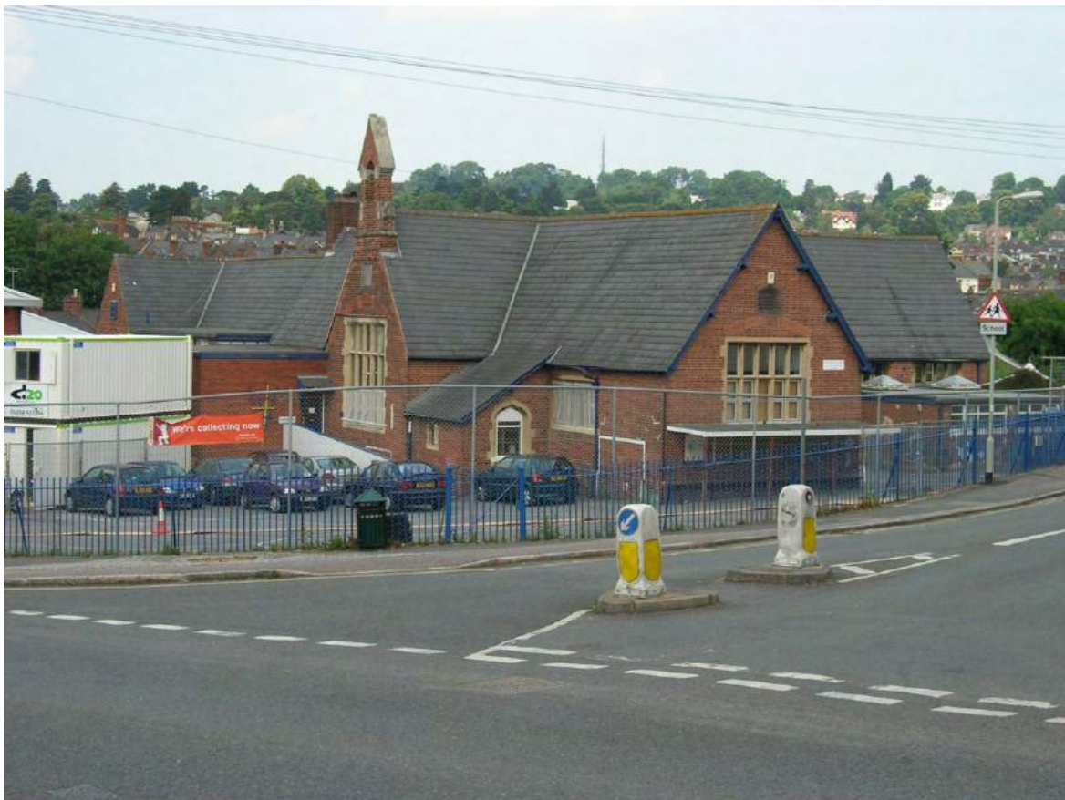
Fig.2 Photograph of the old school from the corner of York Road prior to demolition, July 2006, looking north-east.
