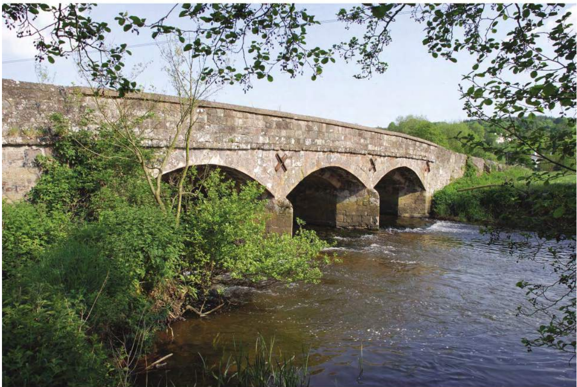
Fig. 11 Stoke Canon Bridge, showing the three river arches of later medieval date, partially hidden behind 19th-century widening.
