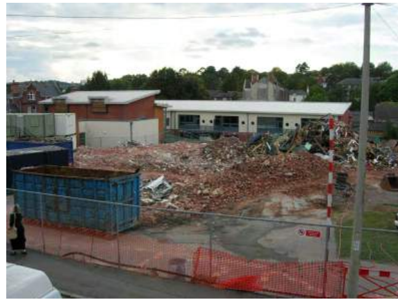
Fig.3 Demolition in progress in September 2006, looking north-west.
