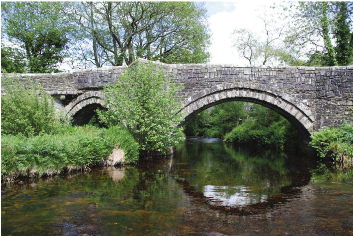
Fig. 15 Huckworthy Bridge, showing one pointed arch and one segmental arch.
